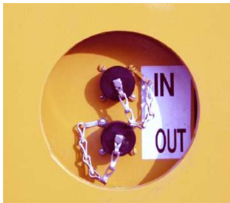
Figure 6.6 - Communication Cable Receptacle.
